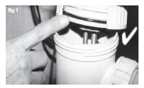
The 'O' ring must be fitted to the control head against the retaining edge before fitting to heater body. Do not rely on locking ring to pull head and body together. Use downward pressure while tightening locking ring. Hand tighten only.
