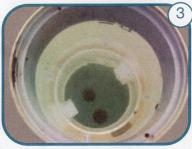
Plug both 2" threaded side ports with 2" plugs and the 1½" balance line port on the pool wall with an expandable or threaded plug. Plug the 2" port(s) in the bottom of the canister.
