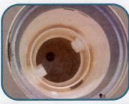
Drain the canister of water using a shop vacuum with a narrow tip or cup. The water level must be below the side ports.
