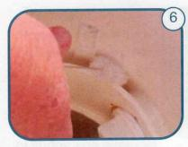
Remove the ring and apply PVC primer and slow/medium set glue, such as IPS Weld-On 705, to ring and canister wall.
